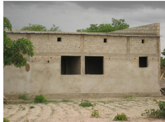
Construction is underway on Phase II of the Medical Center
